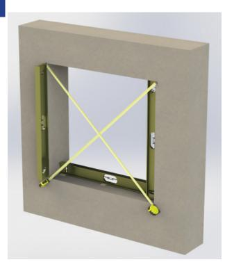
The rough opening should be a minimum  $\frac{1}{2}$ " (but not to exceed 1") wider and taller than the unit. Verify the rough opening is flat, plumb, level, and square. Take diagonal measurements to check for square. The sill beneath the unit must be level for proper unit operation.
